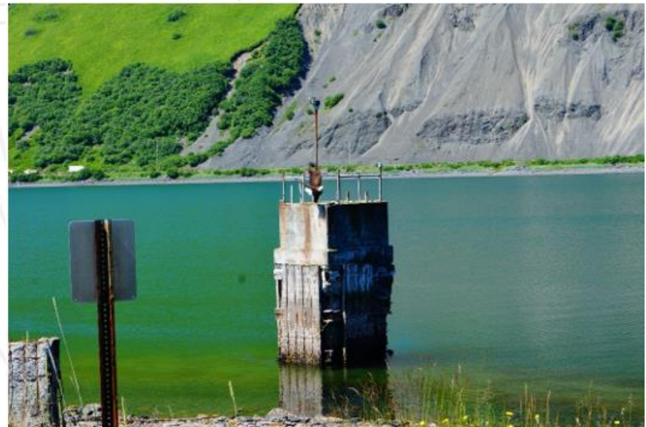
Figure 9. Salt water intake structure, view west.
