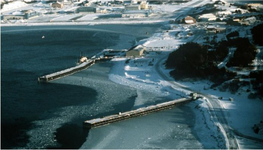
Saltwater intake (barely visible, top middle), 1978 ( above ) and 2016 ( right )
